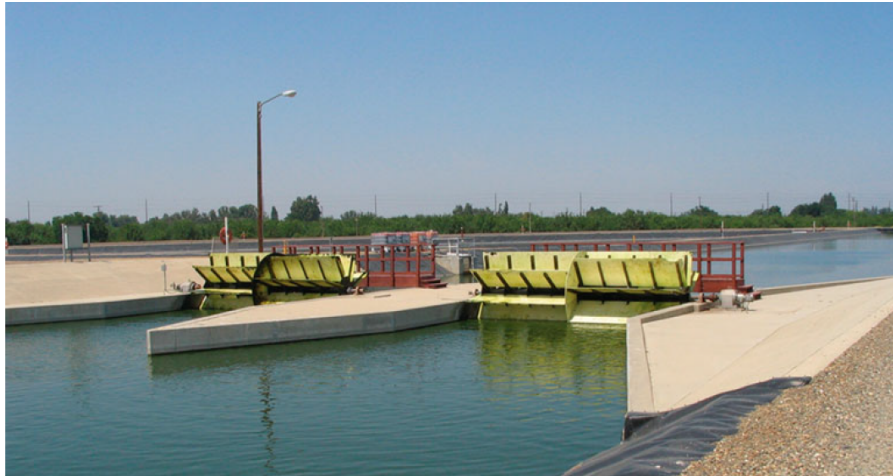
Figure 4: Paddlewheels used in a raceway pond in St Helena and Hilmar California, US [31].
