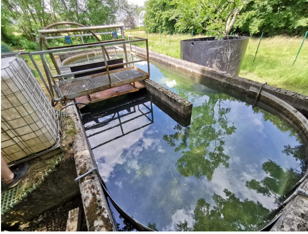
(a) Outlet of the airlift and beginning of the channel.
