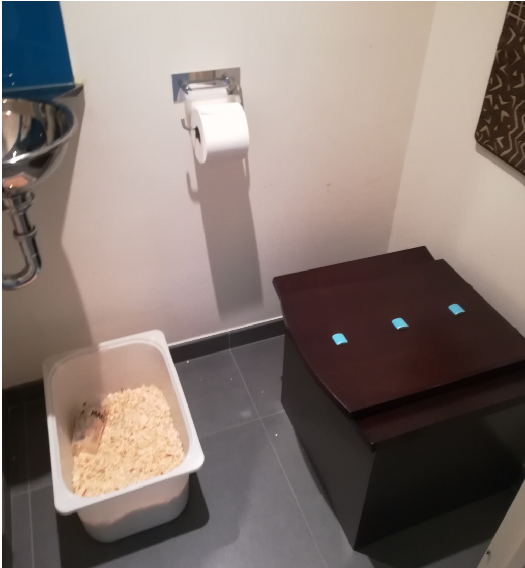
Figure 1 – Exemple of a TLB system inside of a house. Sawdust is available as C-rich cover material.
