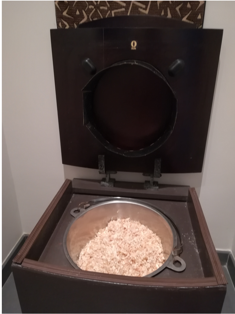
Figure 3 – The collection container is located under the seat. Here, a rubber bib ensures that there is no leakage outside of the container.
