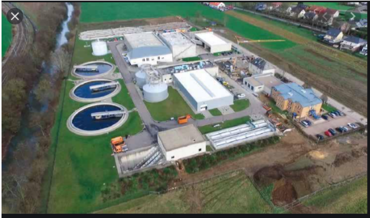
Figure 17: Mersch WWTP overview
