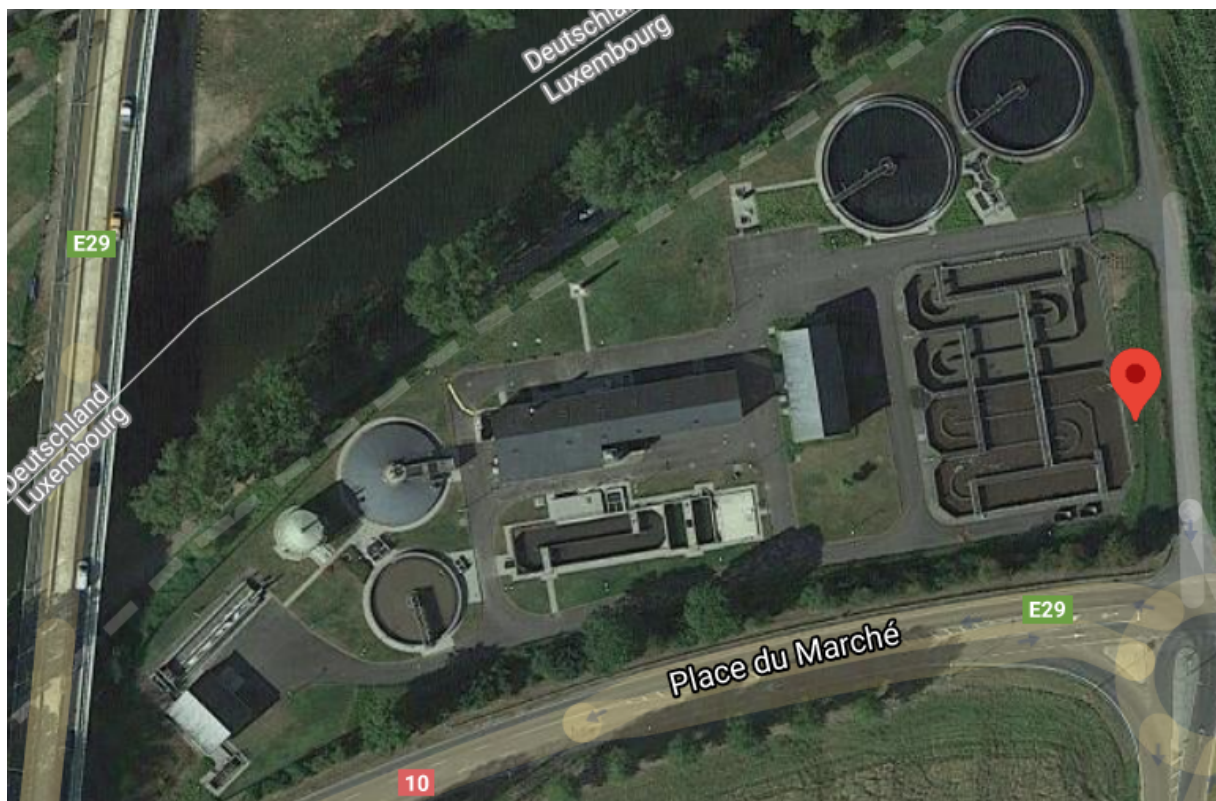
Figure 18: Echternach WWTP overview
