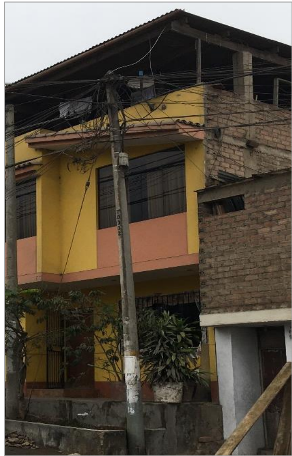
Figure 59: Additional level after awaiting structures 7 years later
