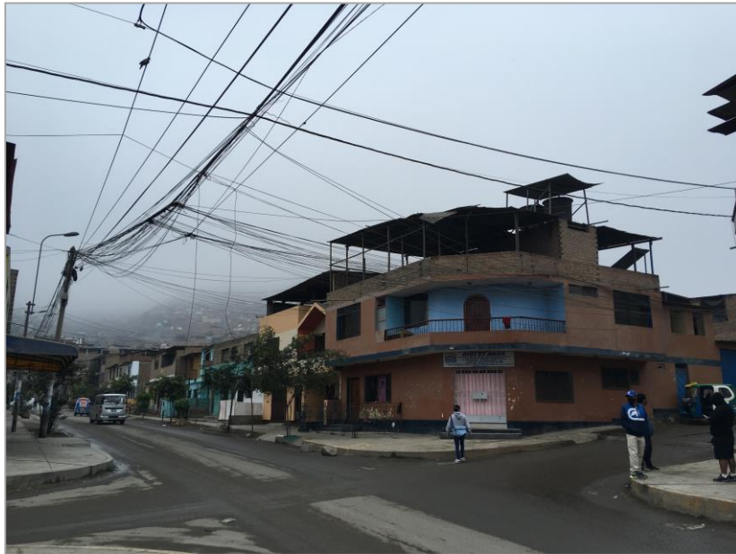
Figure 60: Visual discomfort with electricity wires (Vallecito Alto 2020)
