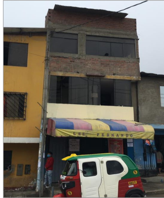
Figure 57: Vertical extension of the house (Vallecito Alto 2020)
