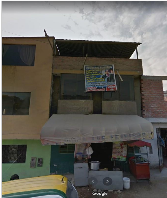
Figure 56: Vertical extension of the house (Source: Google Street View 2013)
