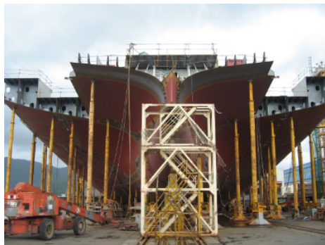
Figure 8. Hull Erection
