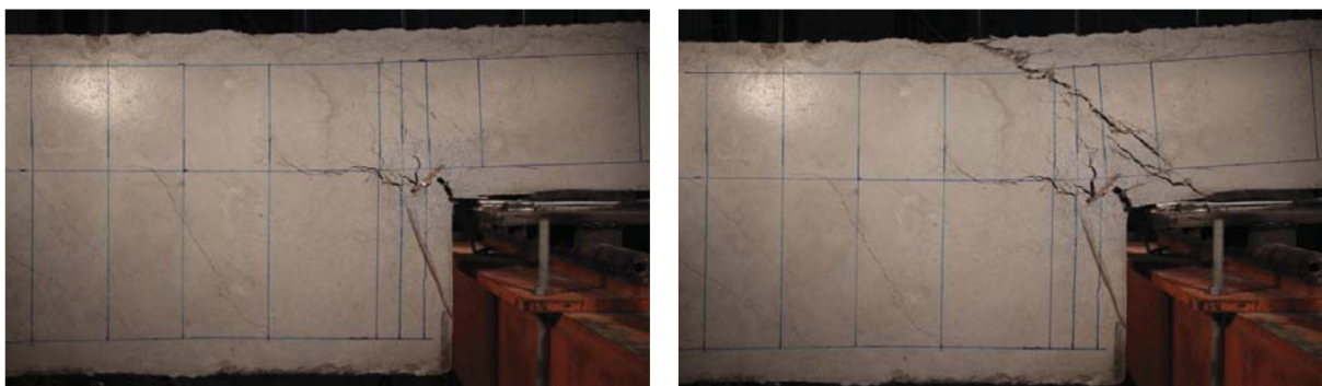
Figure 2.5: Crack patterns on specimen DEB-3.8 (T1) at peak load and ultimate load [15]
