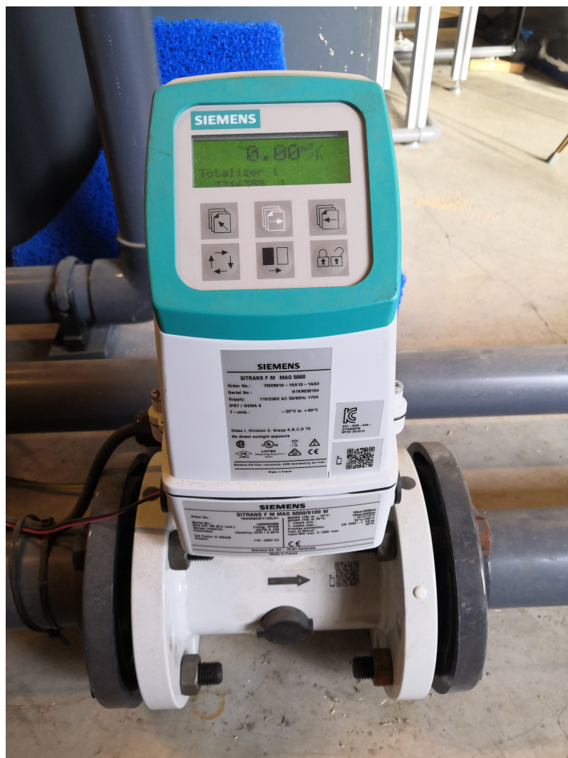
Figure 11: Flowmeter SIEMENS-MAG 5100W.
