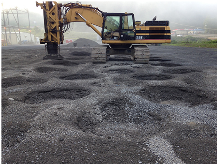
FIGURE 10 – Machine de compaction par impact rapide de grande amplitude [ https://www.terratest.com/ingles/products-rapid-impact-compaction.html ]
