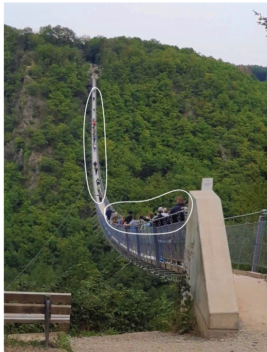
Figure 9: Capture from video post processing showing two groups of pedestrians on the footbridge
