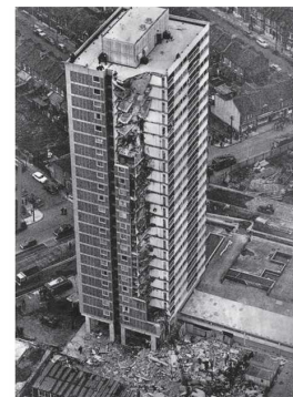
Figure 1.2: Ronan point collapse 2 .
