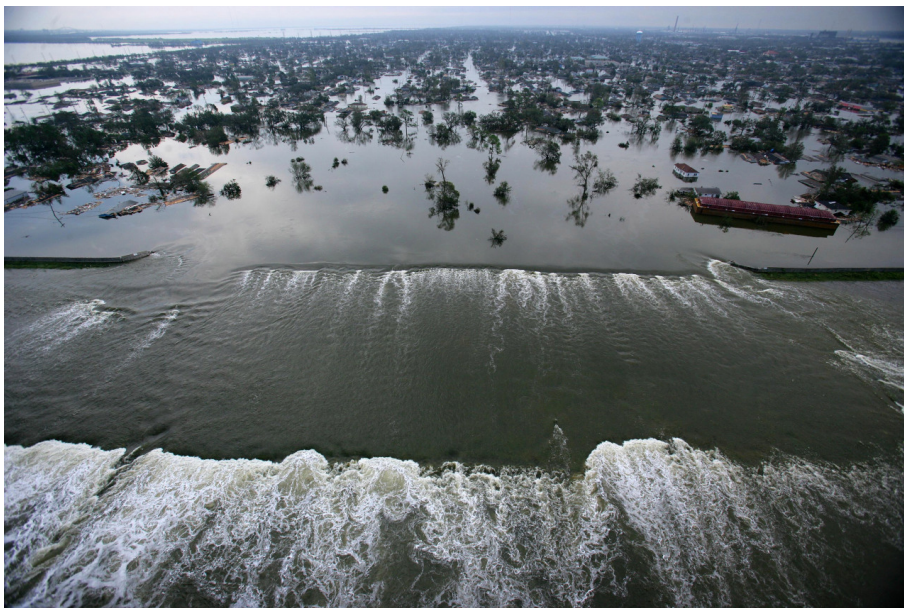
Figure 1.1: Surrounding New Orleans dikes failure (after Hurricane Katrina) caused severe flooding of the city (Hallissy, 2005).
