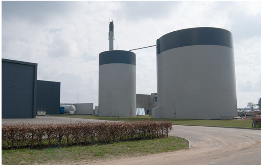
Figure 2.6: Two thermal storage tanks combining for a capacity of 400-500 MWh.
