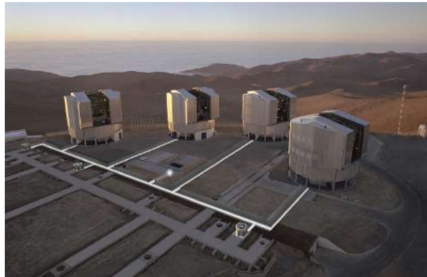
Figure 2.4: Aerial view of the VLT. The four large buildings are the enclosures of the main telescopes. Three auxiliary telescopes can be observed in the foreground. [21]
