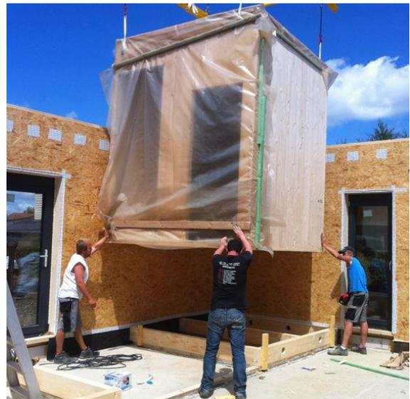
Figure 107 : Pose des modules 3D\_Ncube\_Naturhome.
