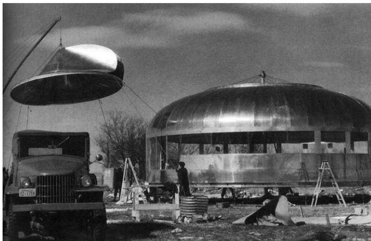
Figure 37 : Dymaxion "Wichita" House\_ Buckminster Fuller\_1945 [Lec19].
