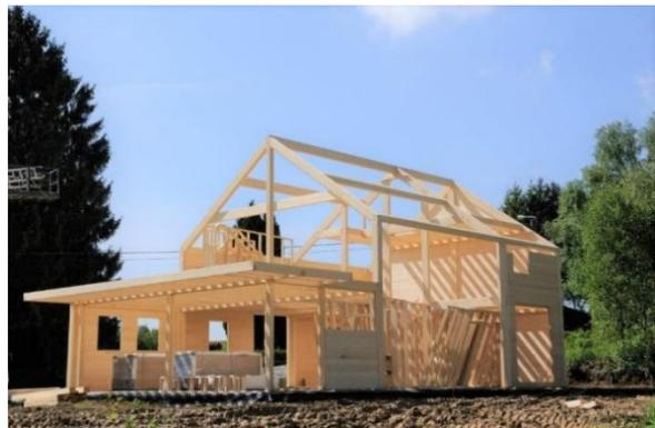
Figure 40 : Construction en poteaux-poutres [Sta21].
