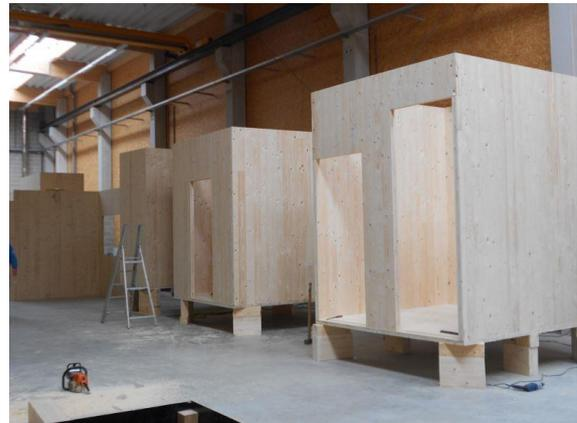
Figure 106 : Construction en atelier\_Ncube\_Naturhome.
