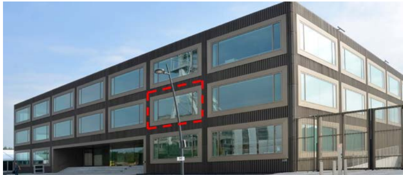
Figure 3-8 EnergyVille 1, Thor Park 8310, 3600 Genk
