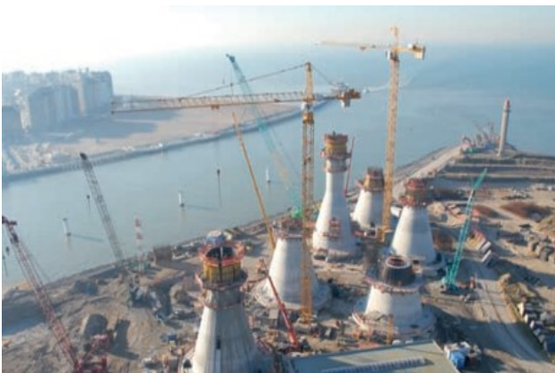
Figure 17. Deep water concept: Thornton Bank [11]
