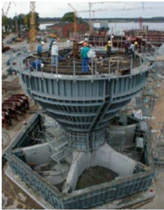
Figure 15. Shallow water concept: Nysted I offshore wind farm foundations [13]
