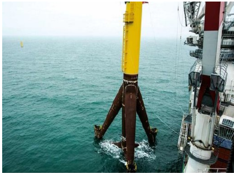
Figure 22. Tripod foundation [22]
