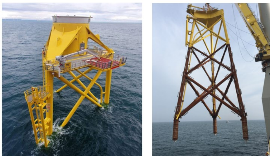
Figure 19. Jacket foundation for three legs with tubular steel piles [16]
