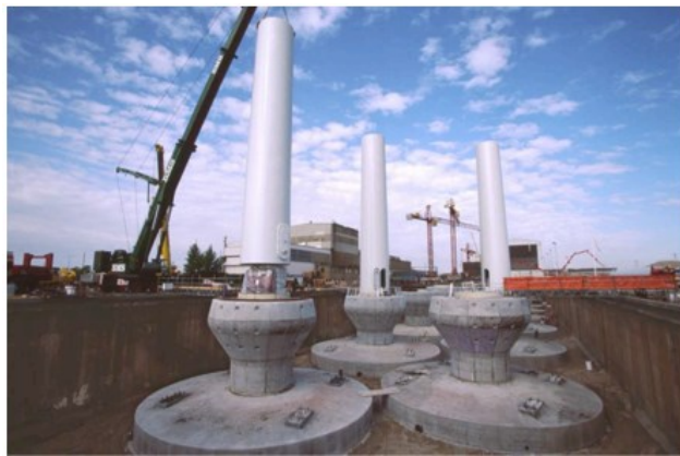
Figure 16. Shallow water concept: Middelgrunden offshore wind farm foundations [14]
