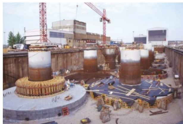
Figure 16. Shallow water concept: Middelgrunden offshore wind farm foundations [14]
