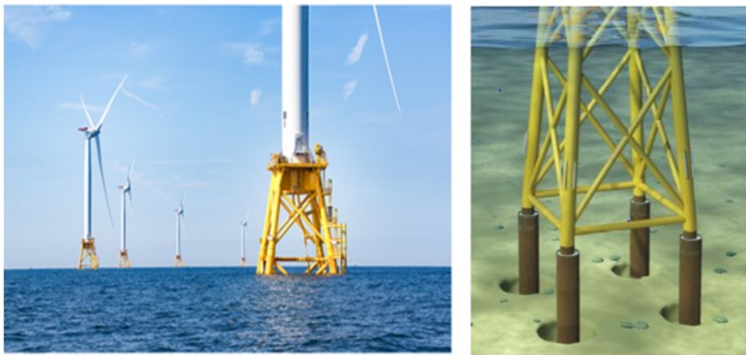
Figure 18. Jacket foundation for four legs with tubular steel piles [15]
