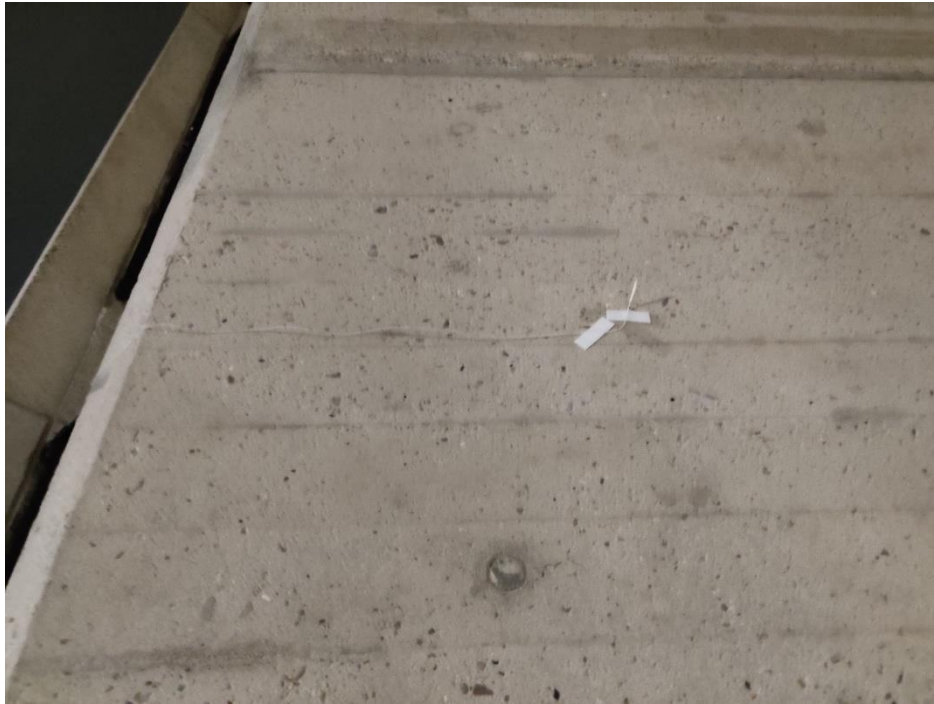
Figure 3-5: Temperature sensor installed outside the building.
