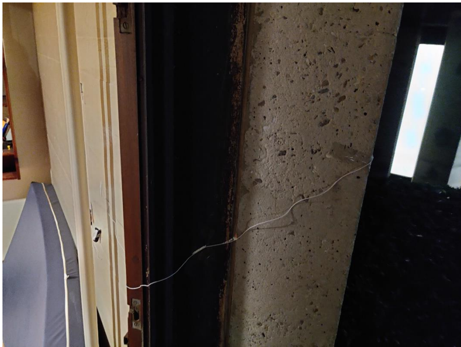
Figure 3-4: External temperature sensor cable passage.
