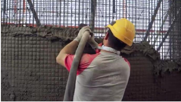
Figure 65 : Gramazio & Kohler, Mesh Mould and In Situ Fabricator, ETH Zurich, 2017.
