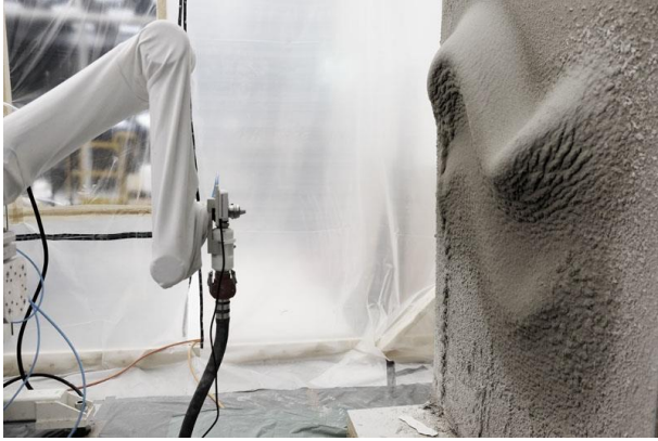
Figure 47 : Gramazio & Kohler, Robotic Plaster Spraying, ETH Zurich, 2018-2022.
