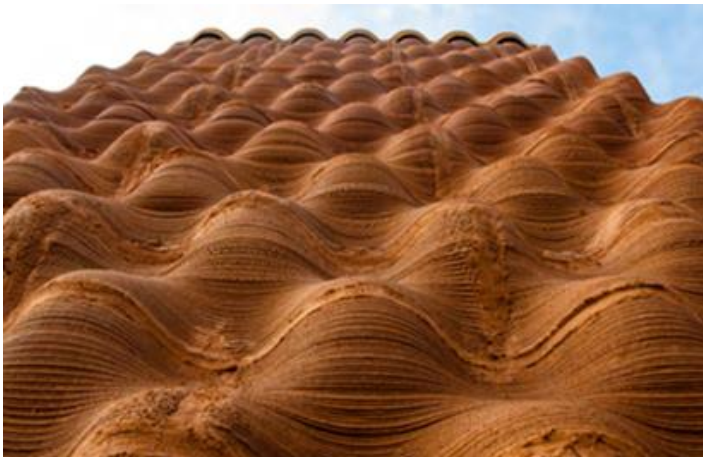
Figure 46 : The Institute for Advanced Architecture of Catalonia (IAAC), Prototype de mur de terre imprimé en 3D, Barcelona, 2017-2018.
