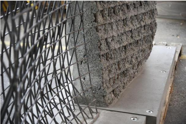
Figure 64 : Gramazio & Kohler, Mesh Mould and In Situ Fabricator, ETH Zurich, 2017.
