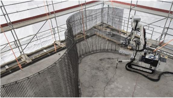
Figure 63 : Gramazio & Kohler, Mesh Mould Prefabrication, ETH Zurich, 2019-2021.
