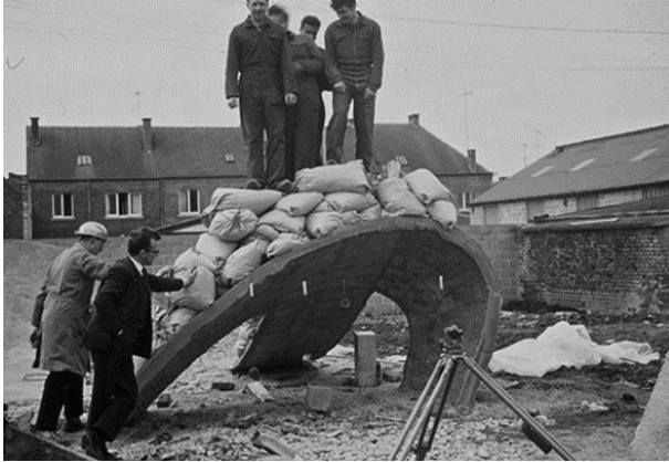
Figure 67 : R. Greish, Test de gunitage, Namur, 1966.
