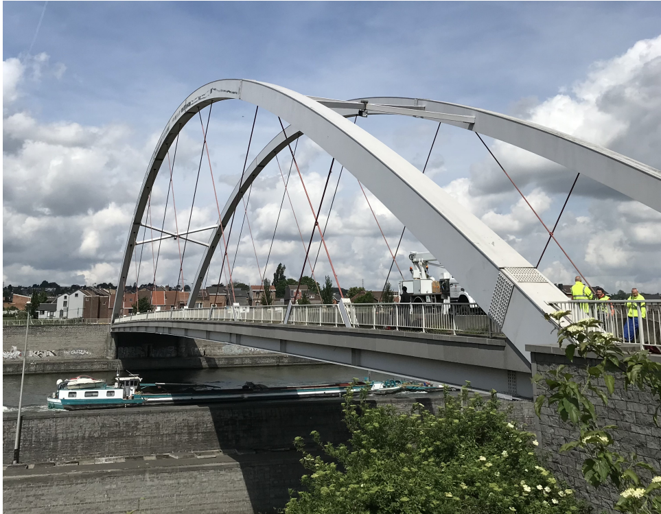
Figure 3.13: Tested cable-stayed bridge, Herstal (Liège).
