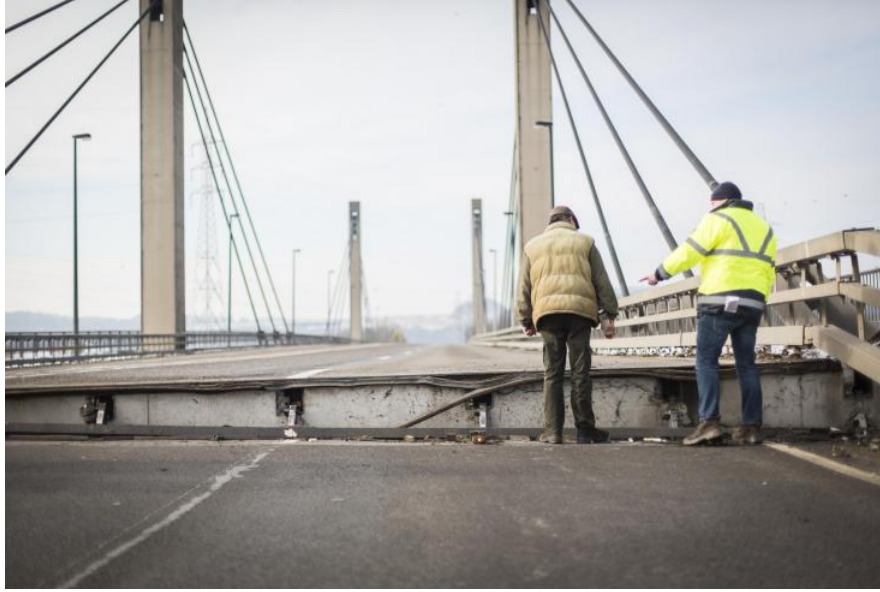
Figure 1.1: Lifting of the Lixhe Bridge (Liège) (URL link , visited in: May, 2022.)
