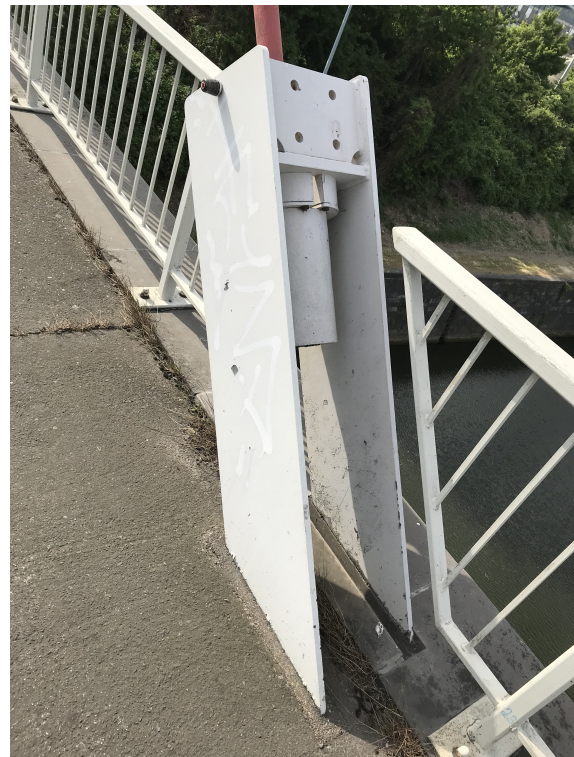
Figure 3.15: Picture of the connector and the anchored support.
