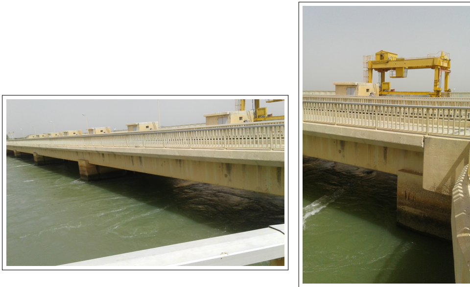
Figure 5: Diama dam, February 2016.
