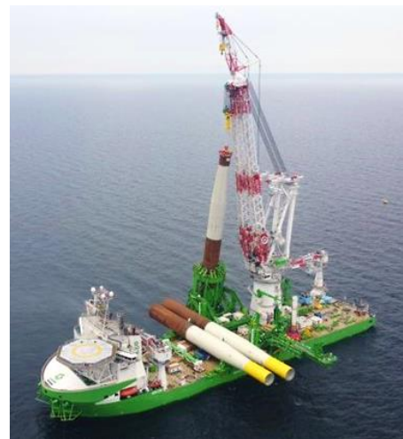
Figure 2: Orion during Installation
