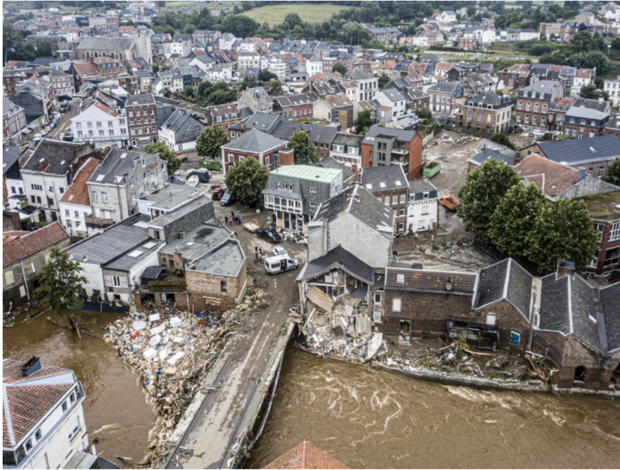
Figure 2.23: Real clogging of the bridge francval
