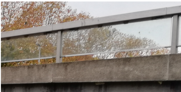
Figure 2.10: Low porosity handrail : thick elements
