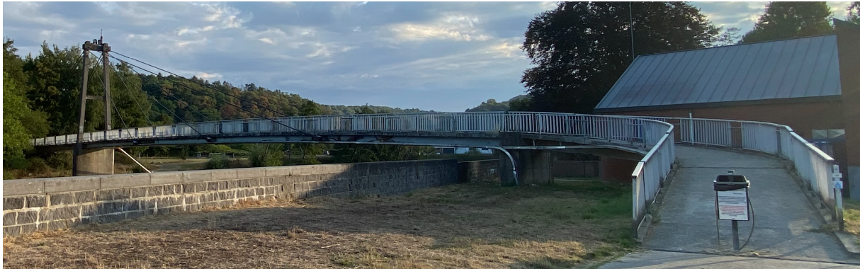
Figure 9: Tilff cable-stayed footbridge.
