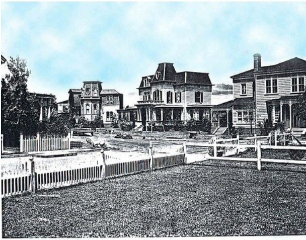
Looking N.W. after grading, paving and landscaping Apr. 1950
