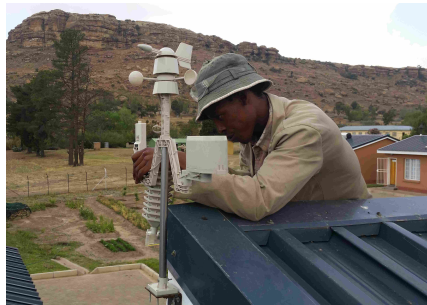
Figure 4.1: Weather station being installed on the roof of a typical clinic in Lesotho
