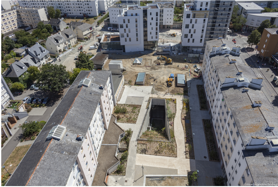
Figure 3.2 – Cleunay station worksite [Personal communication]
