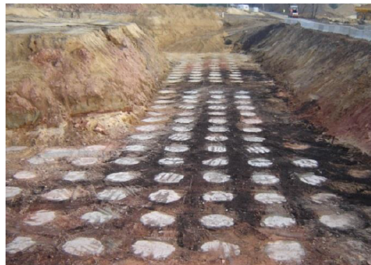
FIGURE 2.20 – Renforcement in-situ [TOPOLNICKI 2016]
