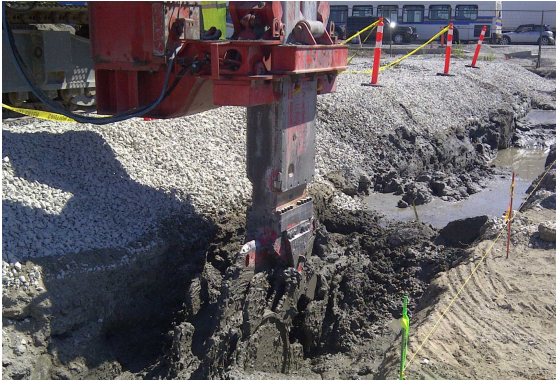
(a) Soil mixing [VIBRO MENARD 2023]
