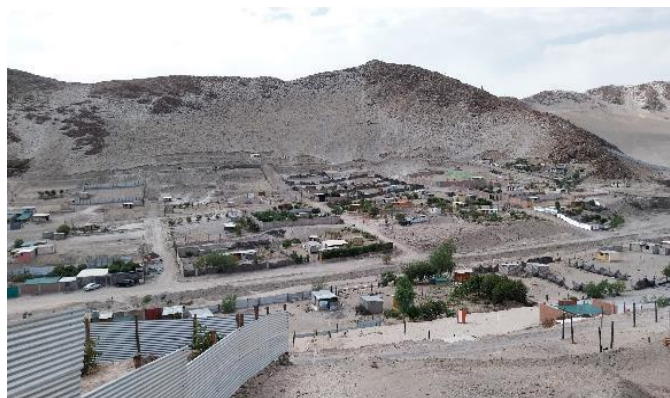
Figure 53: settlement parcels in landslides risk (Photo: H. LE VASLOT)
