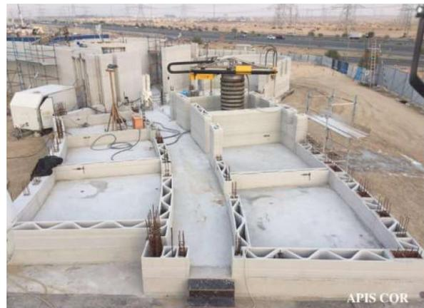
FIGURE 2.5 – L'impression à Dubai [F.P. BOS et al. 2022]
