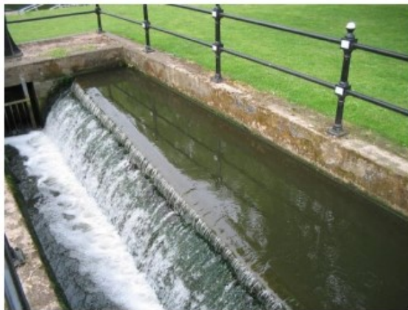
Figure 2.5: Flow over a side weir
