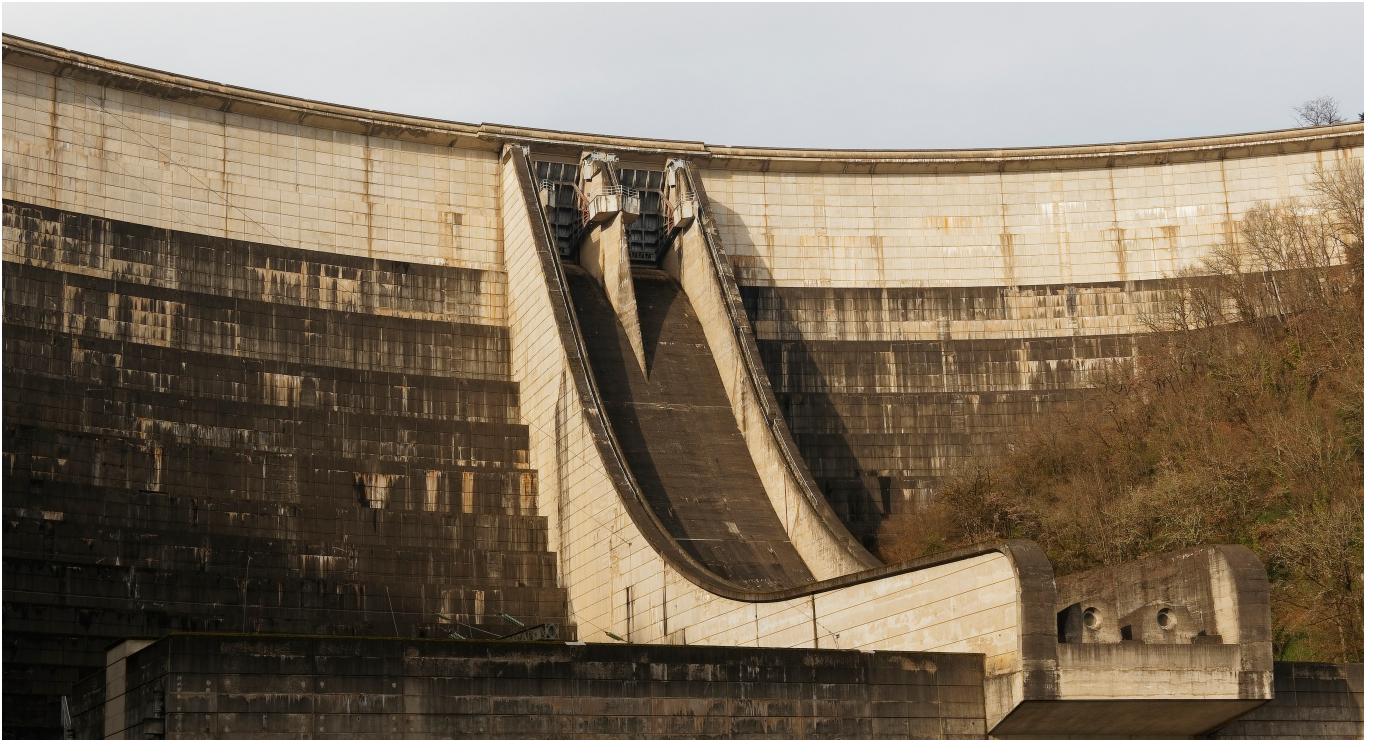
Figure 2.1: Downstream view of the Bort-les-Orgues dam and its gated weir
