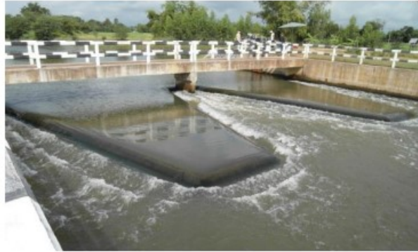
Figure 2.6: Flow over a labyrinth weir
