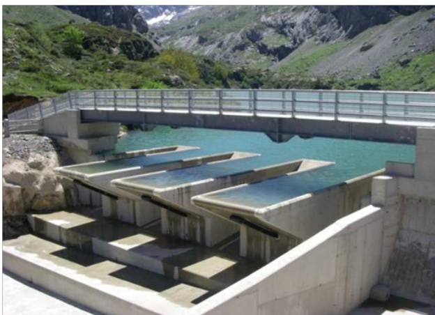
Figure 2.7: Piano Keys weir
