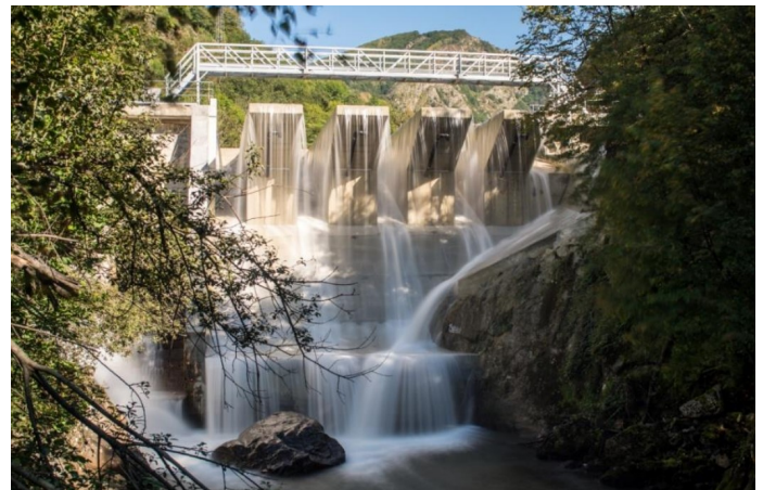
Figure 2.8: Flow over the piano keys weir of Campauleil, France
