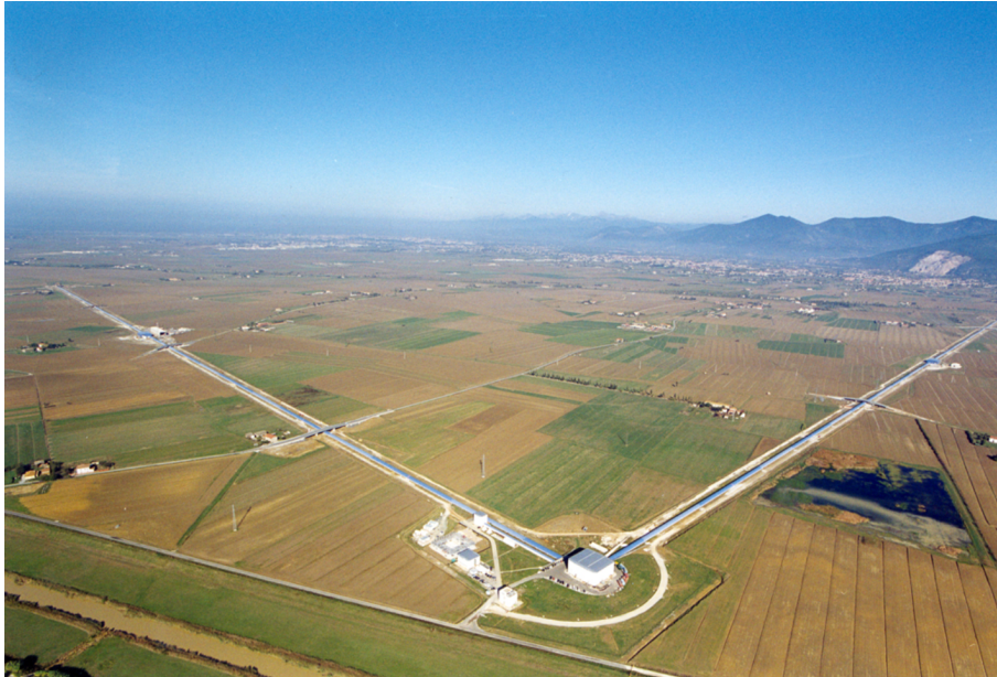
Figure 1.6: The VIRGO observatory, with its two 3-kilometre arms. Located near Pisa, Italy. [16]
