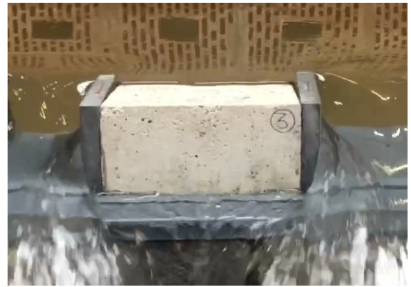
(b) Photo after installation of sealing strip
