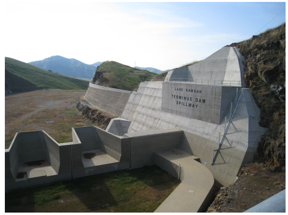
(b) Photo of fuse gates at Terminus Dam in the United States (taken by Chris Austin)
