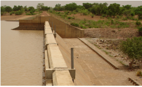
(a) Photo of fuse blocks at Wedbila dam in Burkina Faso (from HydroCoop [2013])
