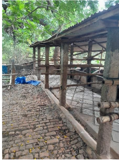
Figure 8: Gutter for the collect of cow urine.
