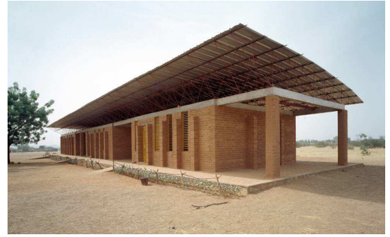
Figure 89 : École primaire de Gando.. © Siméon Duchoud. Source : https://www.kerearchitecture.com/work/building/gando-primary-school-3
