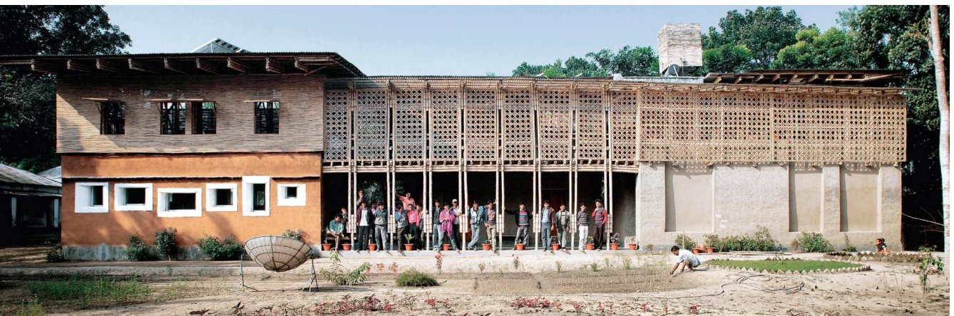
Figure 61 : Projet Desi Training Center d'Anna Heringer. ©Kurt Hoerbst Source : https://arquitecturaviva.com/works/building-desi-rudrapur
