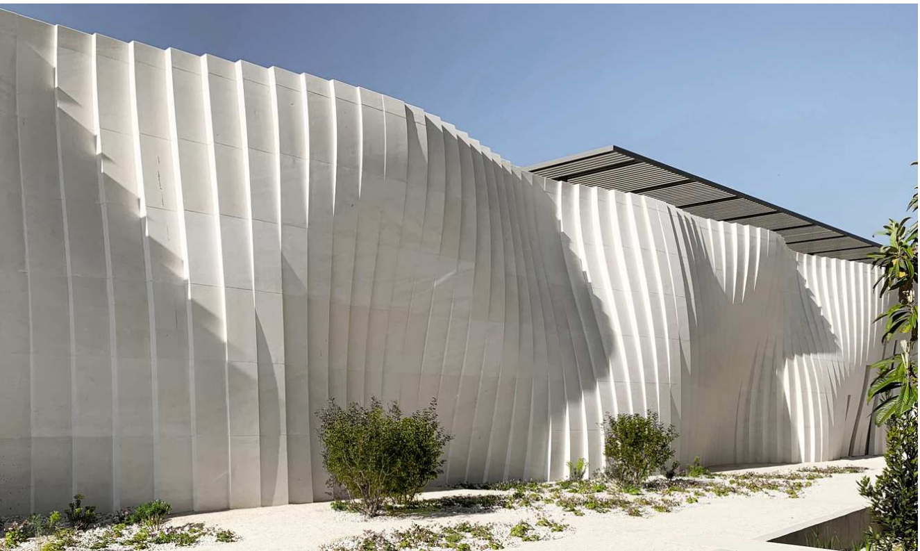
Figure 148 : Le chai Delas, Tain l'hermitage de Carl Fredrik Svenstedt. © Dan Glasser Source : https://www.archdaily.com/933696/delas-freres-winery-carl-fredrik-svenstedt-architecte
