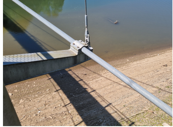
Figure 3.5: Link between the cross-beams and the secondary cables and the hangers.
