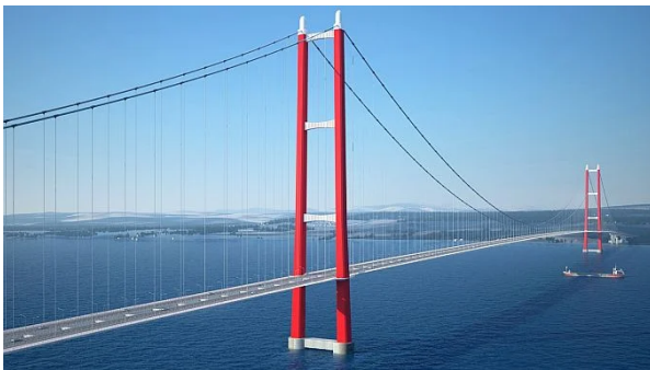
(a)   anakkale Bridge, T  rkiye: the longest suspended bridge in the world, with a span of 2023 m.
