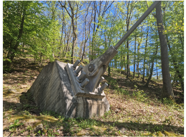
Figure 3.3: Anchorage of the back cables into the ground.
