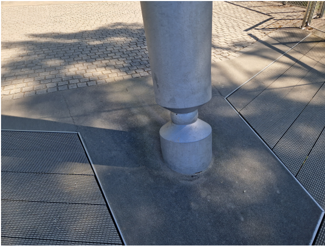
Figure 3.2: Pinned support at the bottom of the pylon.
