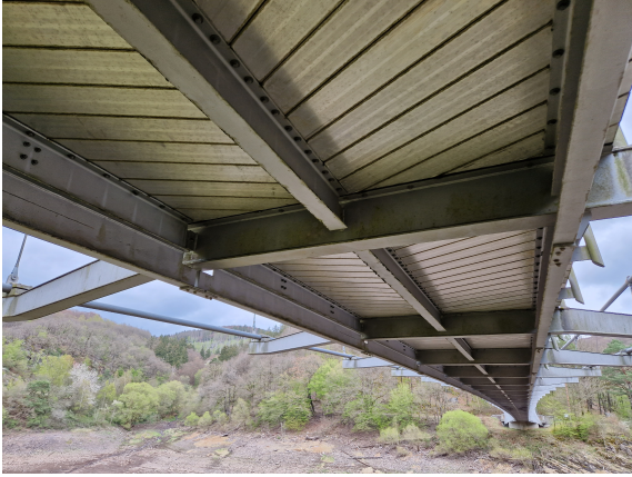
Figure 3.4: Underdeck, with its main components: cross beams and longitudinal beams.
