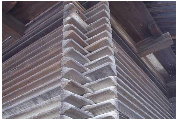
Figure 23: Joint d'angle de construction azekura [81]
