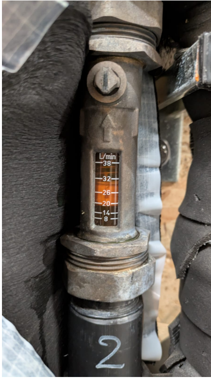
FIGURE A.8: Measured flow rate: 19 L/min
