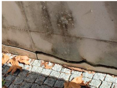
FIGURE 12 – Fissuration du béton (Jesus et al., 2023)
