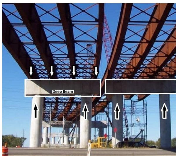
Figure 1: Deep beam in the substructure of a bridge [3]
