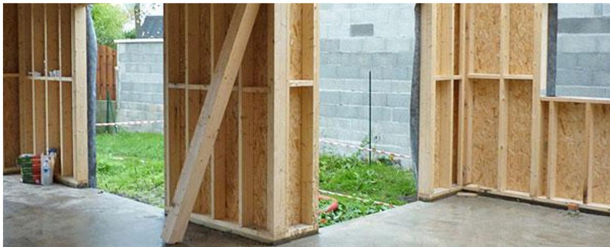
FIGURE 2.4 – VUE DES MONTANTS, DES TRAVERSES, ET DES PANNEAUX DE CONTREVENTEMENT D'UNE OSSATURE BOIS [WWW.LCCB-44.COM]
