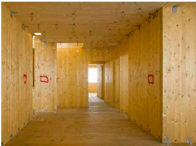
FIGURE 2.26 – MURS ET PLANCHERS EN PANNEAUX MASSIFS EN BOIS [WWW.E-ARCHITECT.CO.UK]
