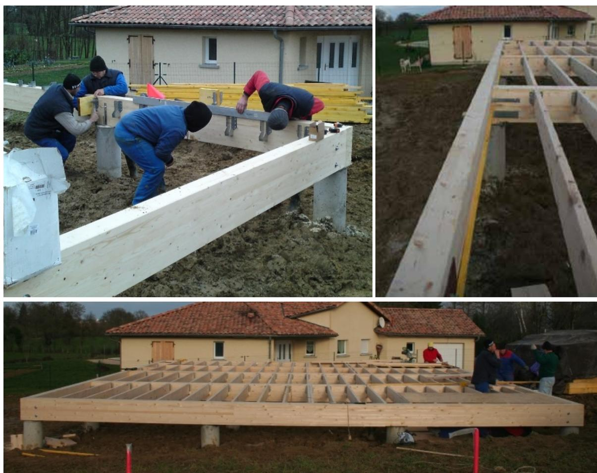
FIGURE 6.9 – MISE EN PLACE DES SOLIVES DE PLANCHER [WWW.NOTREMOB01.CANALBLOG.COM]
