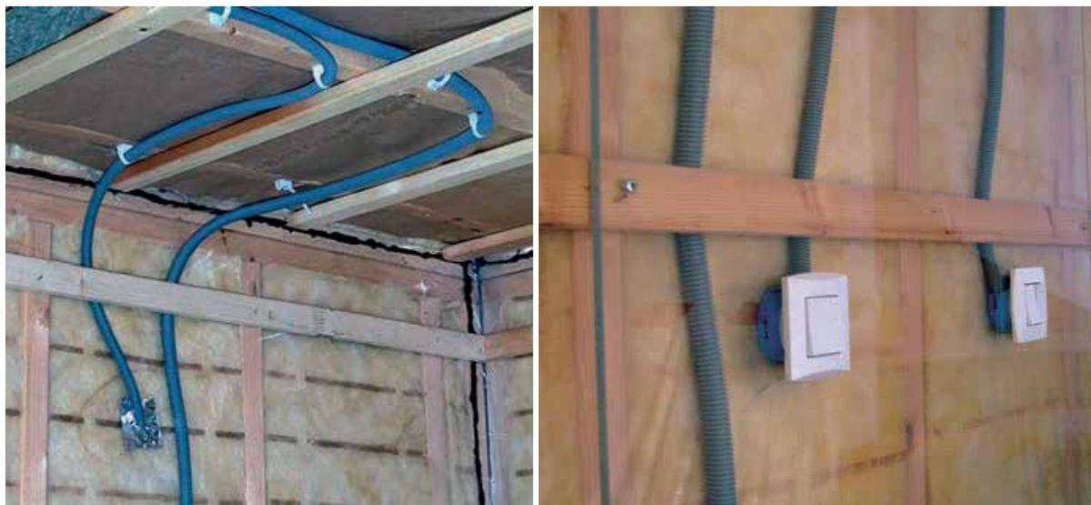
FIGURE 6.27 – FIXATION DE LITEAUX POUR LE PASSAGE DES CÂBLES OU AUTRES [2]
