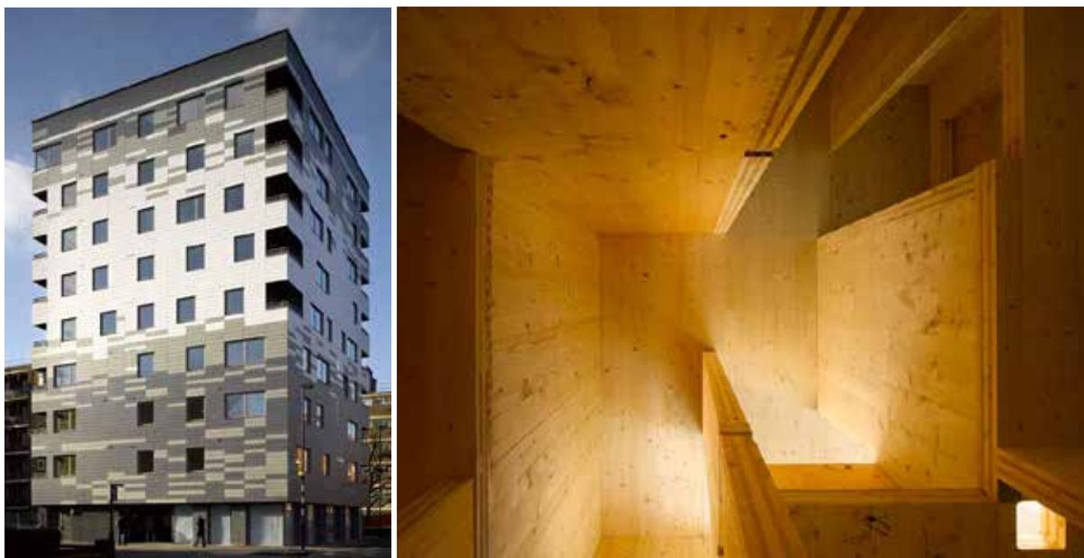
FIGURE 2.21 – BUILDING MURRAY GROVE (STADTHAUS) DE 9 ÉTAGES À LONDRES RÉALISÉ EN PANNEAUX MASSIFS [WWW.E-ARCHITECT.CO.UK]
