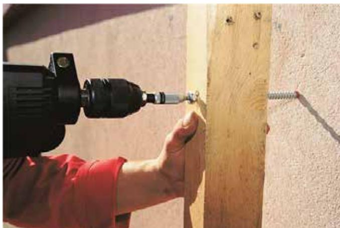
FIGURE 7.9 – FIXATION D'UN MONTANT D'OSSATURE BOIS DANS DE LA MAÇONNERIE [WWW.MEDIA.WURTH.FR]
