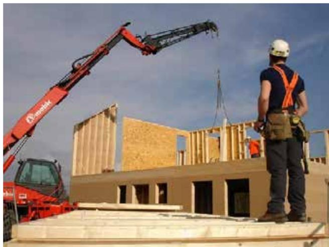
FIGURE 3.3 – MONTAGE D'UNE STRUCTURE OSSATURE BOIS SUR CHANTIER [WWW.GAL.ULYN.NET]
