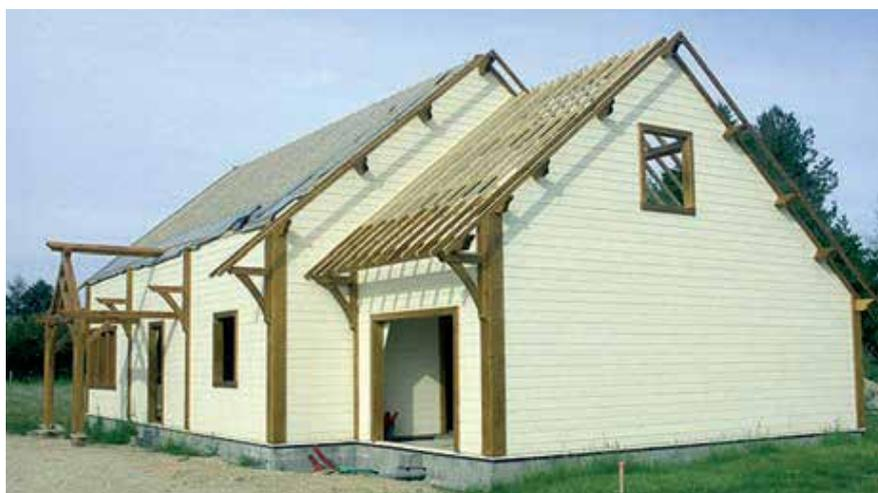
FIGURE 2.14 – EXEMPLE DE REMPLISSAGE QUI PARTICIPE AU CONTREVENTEMENT DE LA STRUCTURE MÊME S'IL N'EST PAS PORTEUR [1]
