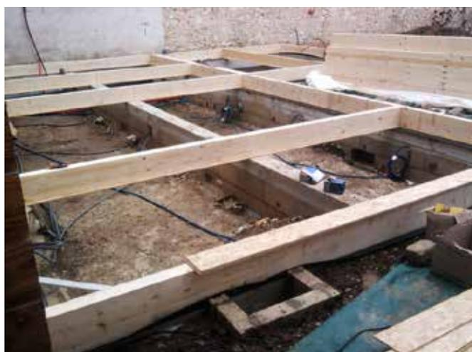
FIGURE 7.7 – SOLIVES DE PLANCHER REPOSANT SUR DES SEMELLES FILANTES [WWW.RENOVATIONECOLOGIQUEAUTOCONSTRUCTION.UNBLOG.FR]
