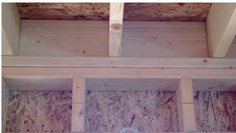
FIGURE 6.18 – SABLÈRE ASSURANT LA LIAISON ENTRE LE MUR ET LE PLANCHER [2]
