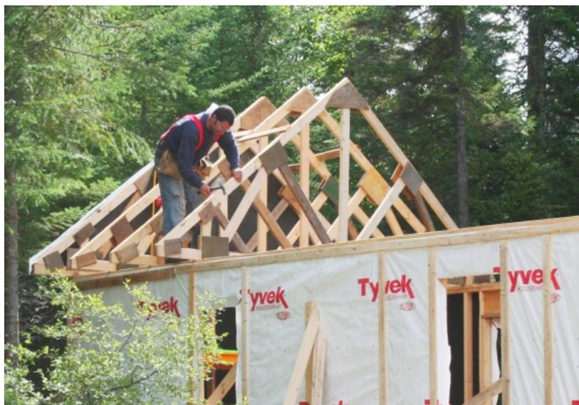
FIGURE 3.5 – MONTAGE DE FERMES DE TOITURE SUR CHANTIER [WWW.DANSNOTREMAISON.COM]
