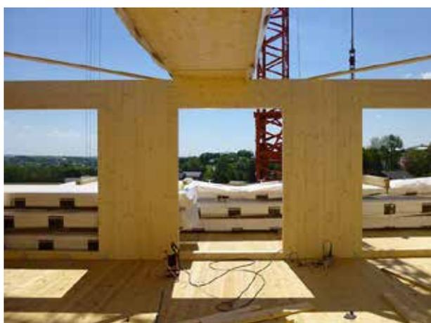
FIGURE 3.8 – MONTAGE D'UNE STRUCTURE EN PANNEAUX MASSIFS SUR CHANTIER [WWW.TIMBERTEAM.NET]
