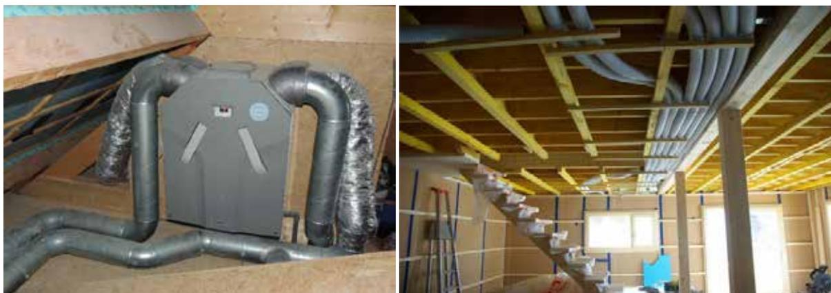
FIGURE 6.28 – VMC DOUBLE FLUX [WWW.CONSTRUCTION-MAISON-OSSATURE-BOIS.INFO, WWW.A133.IDATA.OVER-BLOG.COM]
