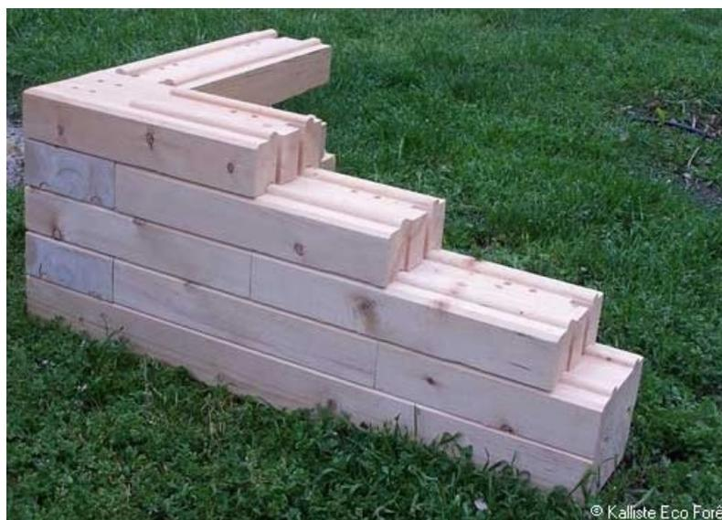
FIGURE A.13 – MONTAGE DES PARPAINGS EN BOIS MASSIF [KALLISTE ECO FORÊT]
