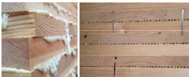
FIGURE 2.24 – COLLAGE (À GAUCHE) ET CLOUAGE (À DROITE) DES LAMES DE BOIS [WWW.SMITHANDWALLWORK.COM]
