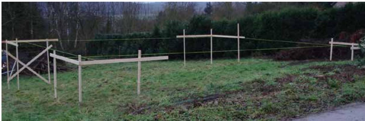
FIGURE 1.9 – CHAISES DÉLIMITANT L'EMPLACEMENT D'UNE CONSTRUCTION [WWW.CONSTRUCTION-MAISON-OSSATURE-BOIS.INFO]
