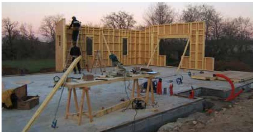
FIGURE 6.4 – MONTAGE D'UNE OSSATURE BOIS DIRECTEMENT SUR UNE DALLE DE SOL EN BÉTON
