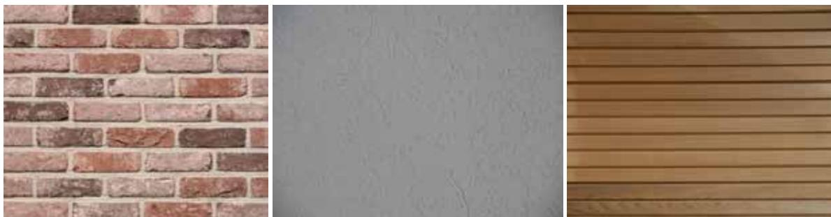
FIGURE 1.8 – DIVERSES POSSIBILITÉS D'ENVELOPPE EXTÉRIEURE (BRIQUE DE PAREMENT [WWW.BE.ALL.BIZ], CRÉPI [WWW.IMAGES.DOCTISSIMO.FR], BARDAGE EN BOIS [WWW.WOODSTOXX.BE])
