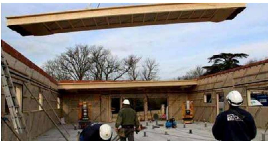
FIGURE 3.4 – MONTAGE D'ÉLÉMENTS DE PLANCHER SUR CHANTIER [WWW.GUIDEBATIMENTDURABLE.BRUXELLESENVIRONNEMENT.BE]
