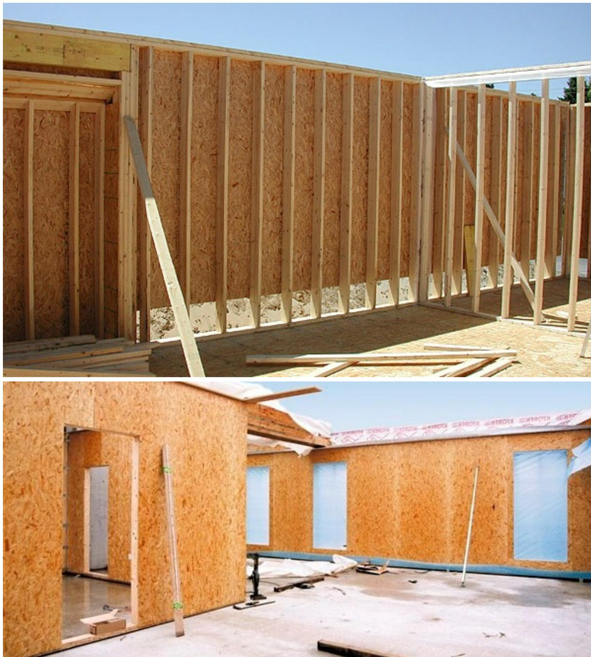
FIGURE 6.14 – PANNEAUX POSÉS SUR UN SEUL CÔTÉ OU MURS FINALISÉS [WWW.MONISOLATIONEKOLOGIQUE.COM, WWW.SAINTHIMAT.COM]
