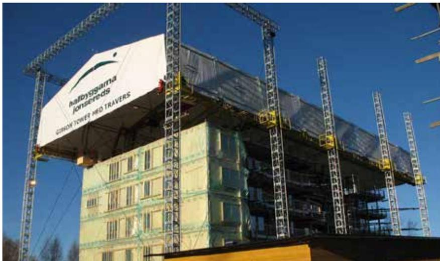
FIGURE 2.30 – STRUCTURE DE PROTECTION D’UN SITE DE CONSTRUCTION [FPIINNOVATIONS]
