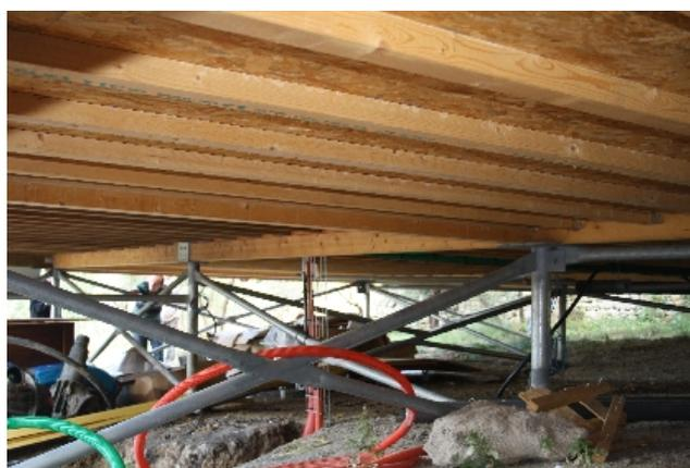
FIGURE 6.5 – PLANCHER EN BOIS SUR MICROPIEUX (AÉRÉ PAR EN DESSOUS) [WWW.BTSTC-LAMOUR.ORG]
