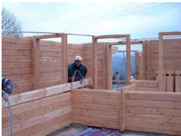
FIGURE 3.7 – MONTAGE D'UNE STRUCTURE EN BOIS MASSIF EMPILÉ SUR CHANTIER [WWW.MAMAISSONMESTRAVAUX.COM]
