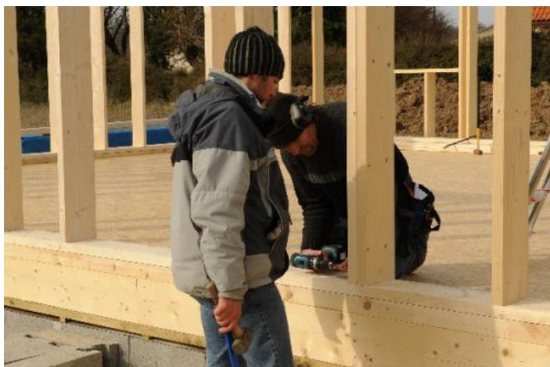
FIGURE 6.13 – ASSEMBLAGE DES CADRES POSÉS SUR UNE LISSE BASSE ELLE-MÊME FIXÉE AU PLANCHER [10]
