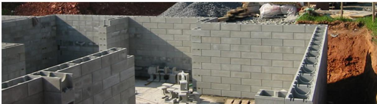
FIGURE 1.2 – FONDATIONS EN MURS ARMÉS (ARMATURES + BÉTON COULÉ ENTRE LES BLOCS CREUX)
