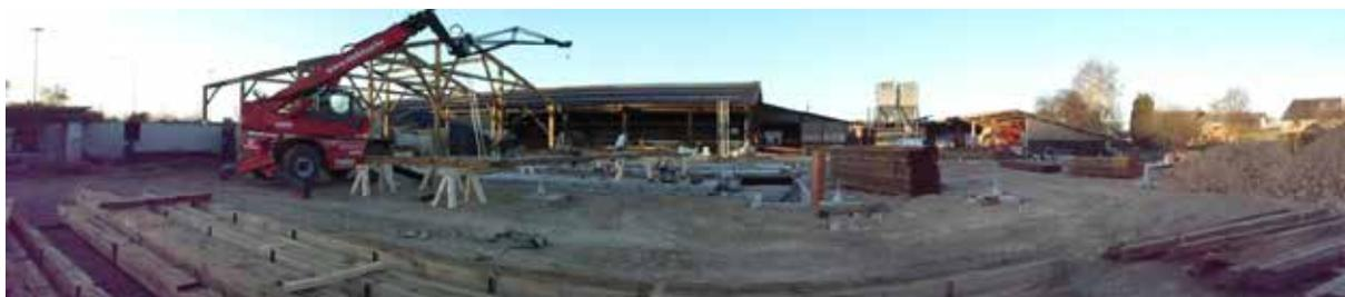
FIGURE 3.6 – MONTAGE D'UNE STRUCTURE POTEAUX/POUTRES SUR CHANTIER [WWW.MYBESTCV2.CO.IL]
