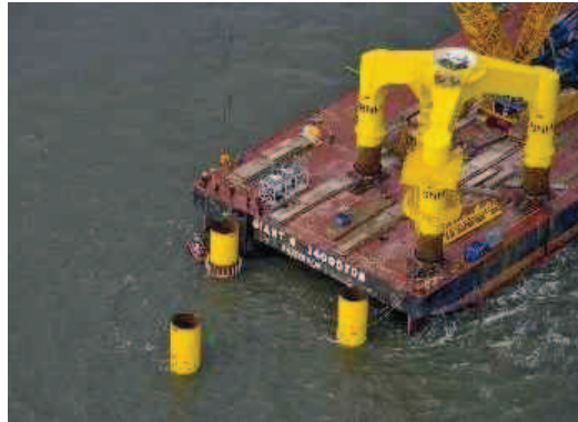
Figure 20: Installation of the transition piece of the tri-pile foundation at BARD 1 offshore 20
