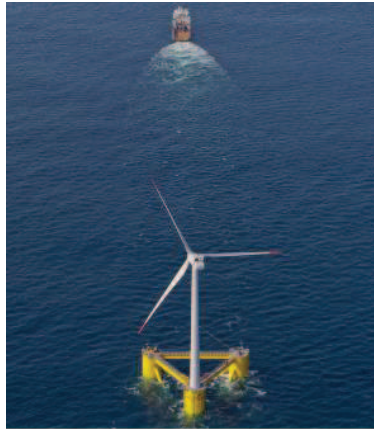
Figure 24: Towing out of WindFloat 24
