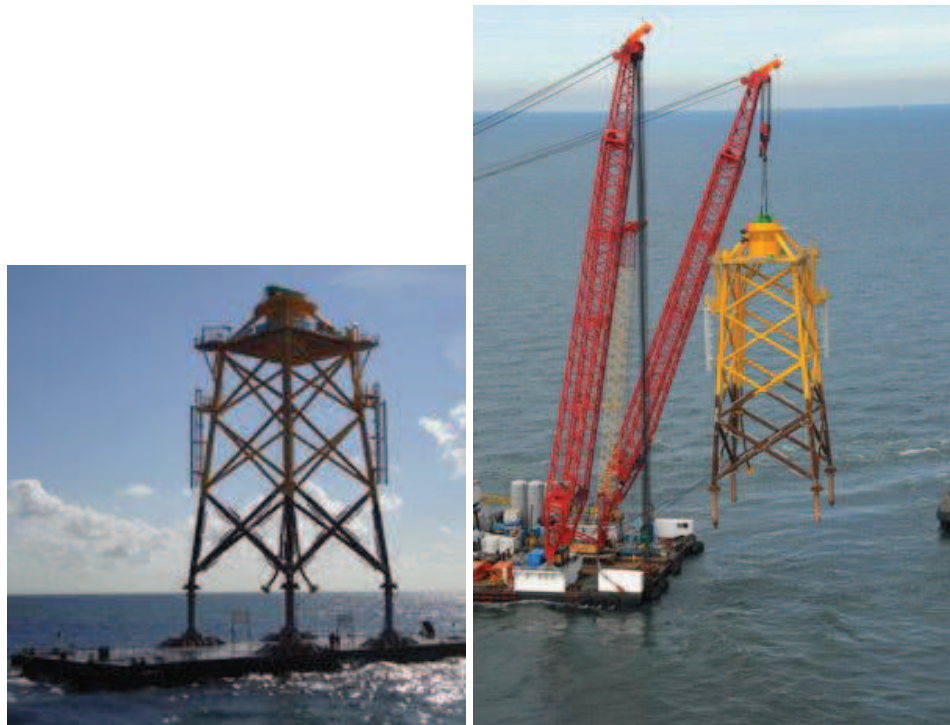
Figure 18: Transport and installation of the jacket 18
