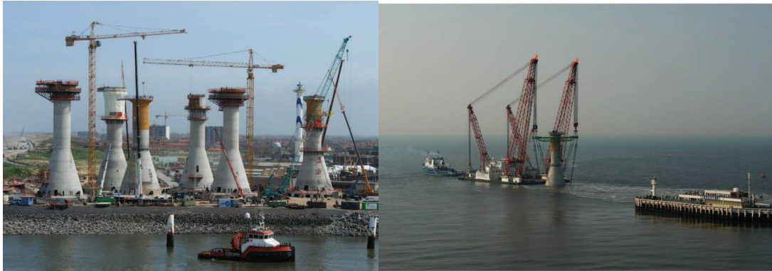
Figure 16: Construction and transport of the gravity based foundations on the Thornton Bank project 16
