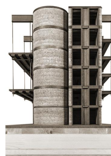
**Figure 124 : Steel House, structure en acier et pisé, Boltshauser Architekten, Lausanne, 2016-2017.** Straube, S. L. (s.d.). Case Study Steel House [photographie]. Boltshauser Architekten. <https://boltshauser.info/projekt/case-study-steel-house/>
