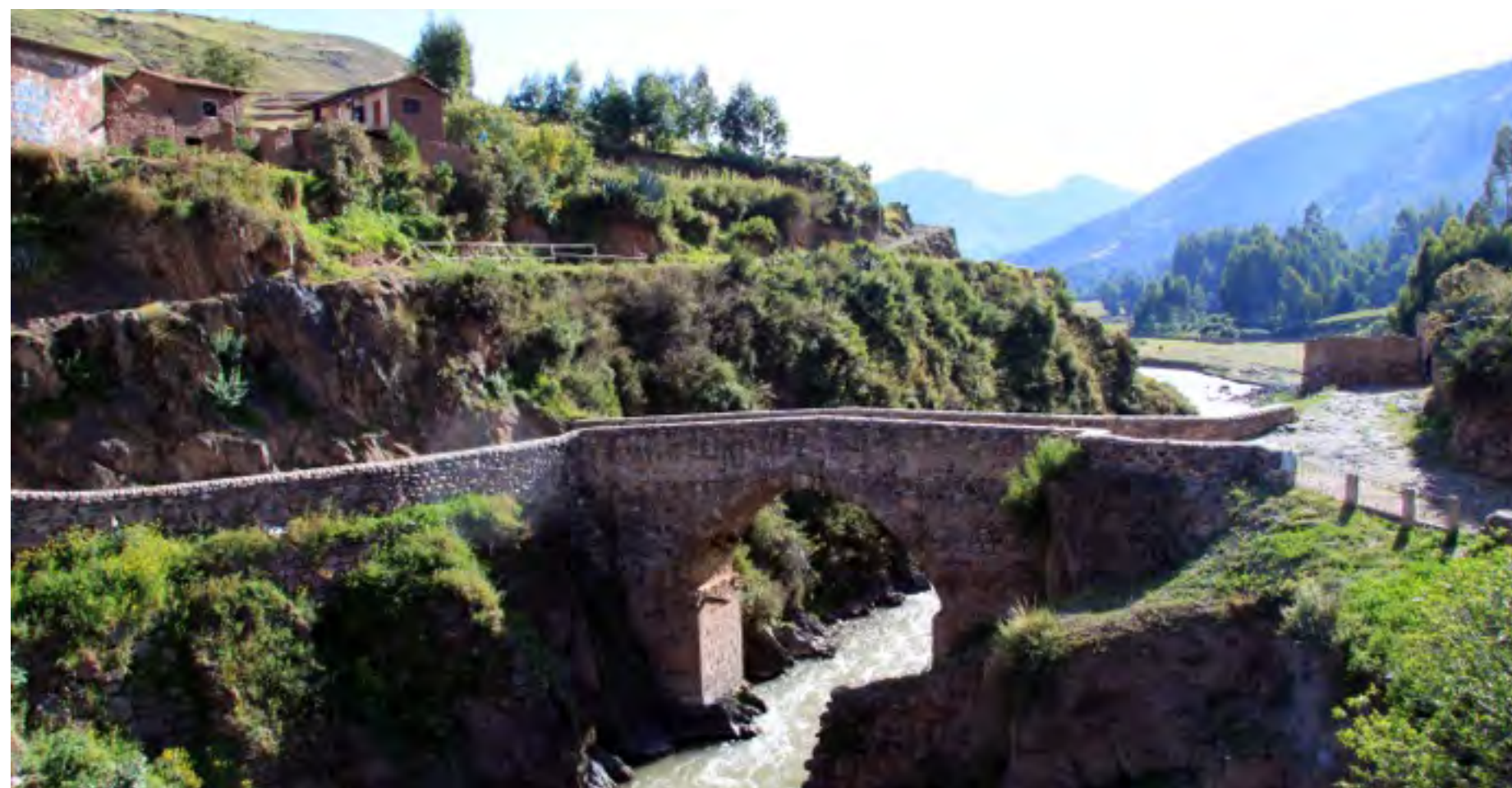
Checacupe, pont colonial
