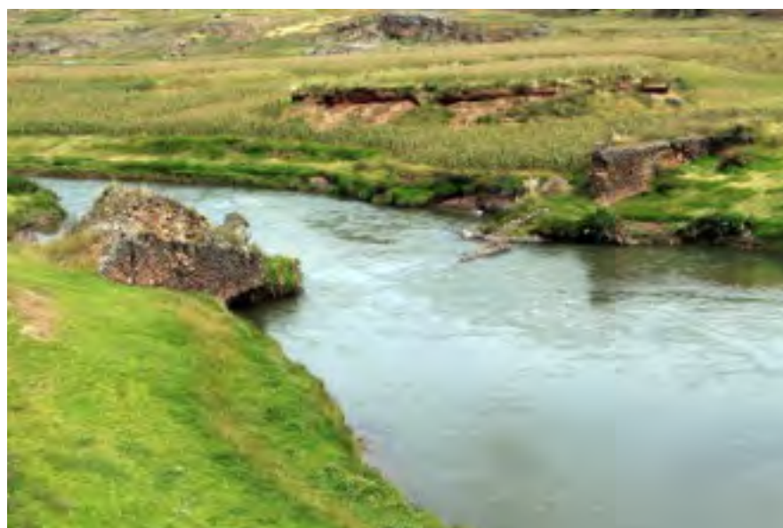
7-2, pont colonial effondré
