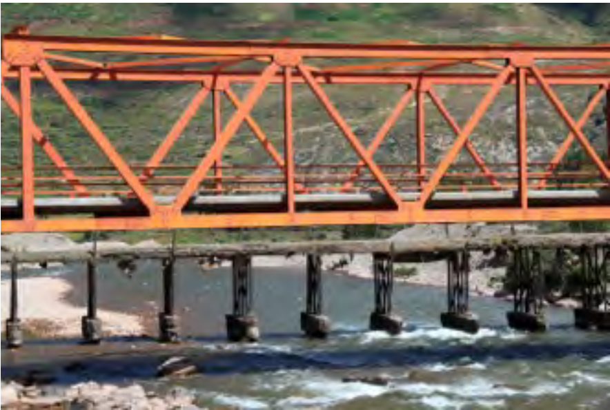
8-1, Combapata, pont contemporain
