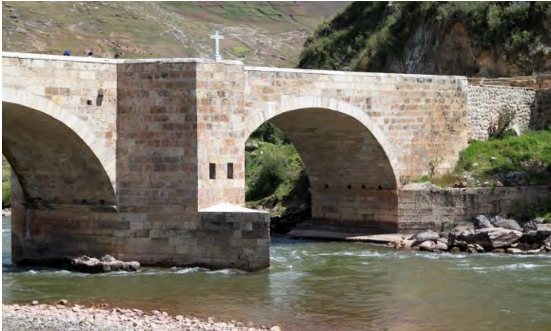
8-1, Combapata, pont colonial
