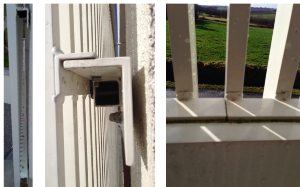
Figure C.1 – Real view on site of cylinders fixation
