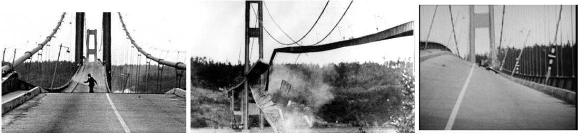
Figure 1.3 – Tacoma bridge collapse (1940), from Vortex Induced Vibration/Galloping combination [3]
