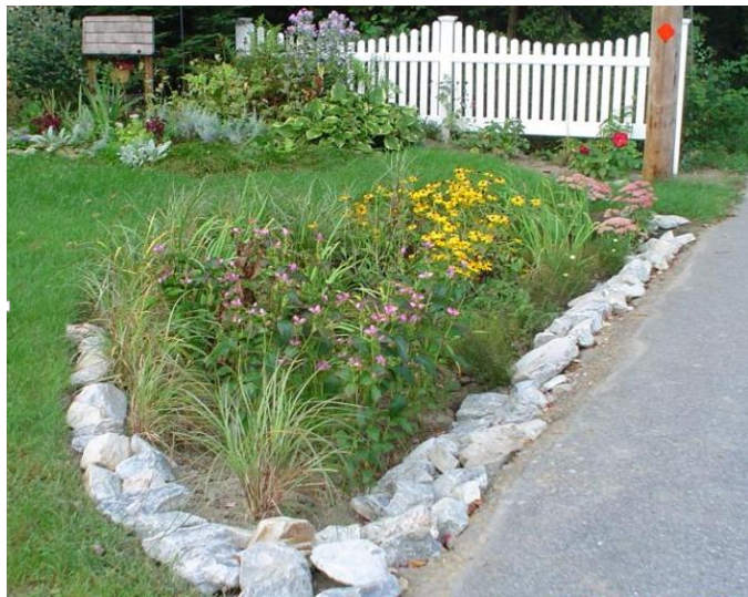
Figure 2: Example of bioretention cell [2]
