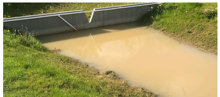
(b) Triangular weir as a control mechanism
