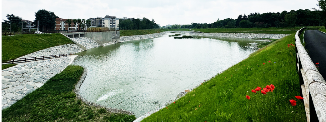
Figure 1.3: Detention pond for the Seveso torrent in Milan [30]
