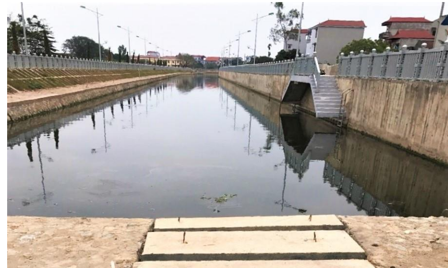
Figure 4.15 – Infrastructure supportant le canal principal (Source: cliché issu de l'enquête, 2017)
