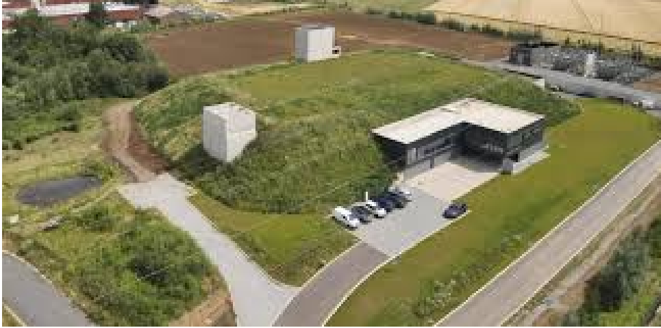
Figure 1.1: The BeCOVER aerodynamic test center infrastructure in Herstal. [3]
