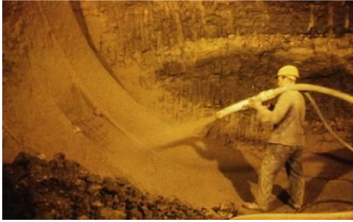
(a) Projection of shotcrete.
