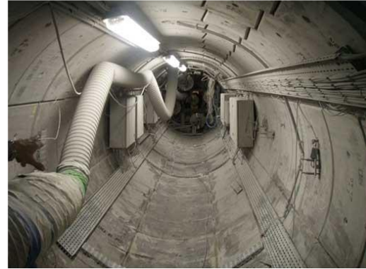
(b) Concrete precast elements.
