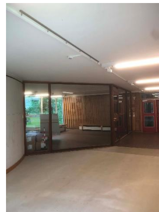
Figure 51 - Photo de la zone 6
