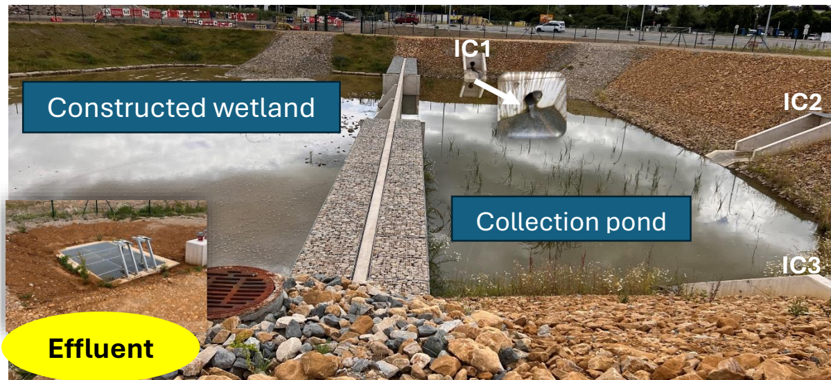
Figure 4. Overview of the Raemerich stormwater treatment system, showing inlet structures (IC1-IC3), the collection pond, and the VF CW.
